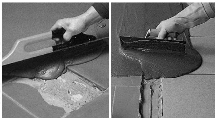
Figure 6. Cementitious levellings
