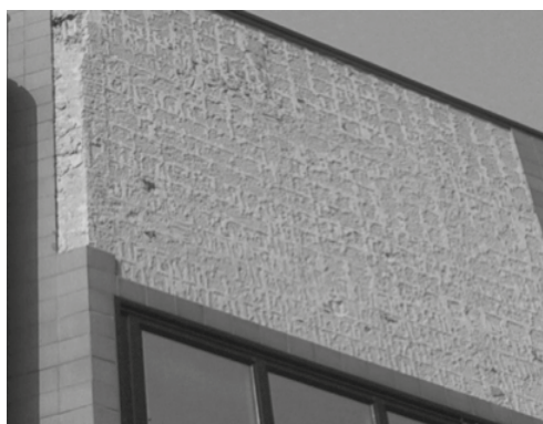
Figure 12. Tiles detaching
