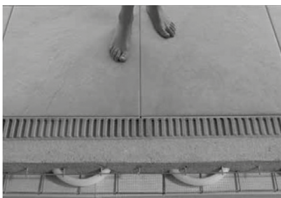
Figure 7. Stratigraphy of a heating screed
